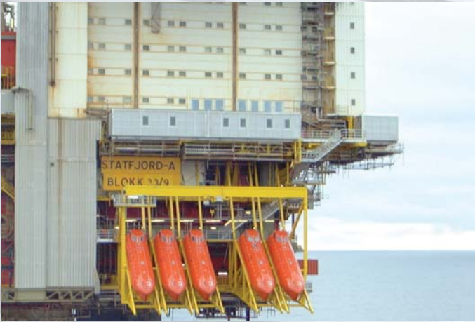
STATFJORD A MODULES AFTER INSTALLATION.
