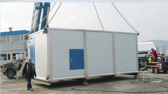
TESTLIFTING OF STATFJORD A – CONTROL ROOM MODULE.
