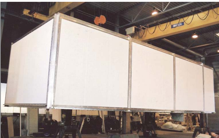
STATFJORD A MODULE AFTER WALL ASSEMBLY.
