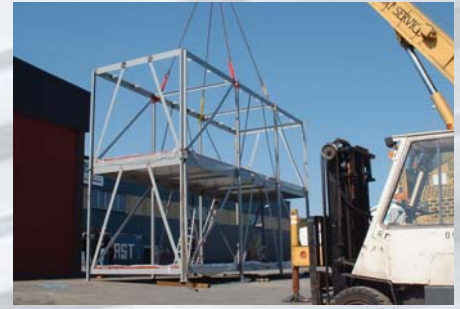
STRUCTURAL ASSEMBLY OF OFFICE MODULES LB 4000 (MILD STEEL)
