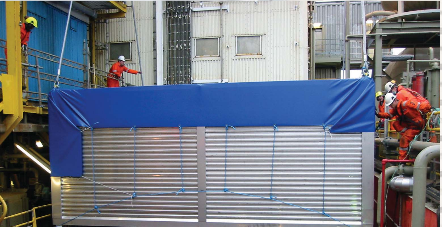
4 STOREY OFFICE BLOCK INSTALLED DECK BY DECK AT AT STATFJORD A.
