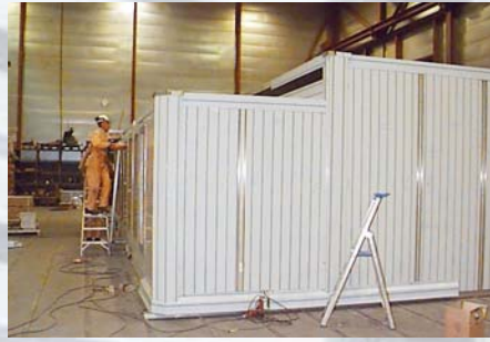
STATFJORD A – WELL BEEING CENTRE. TEST ASSEMBLY OF FLAT PACK DELIVERY.
